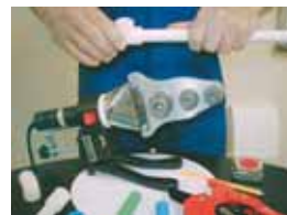
3; Within the allowed time interval, connect the pipe and the fitting (do not twist.)
