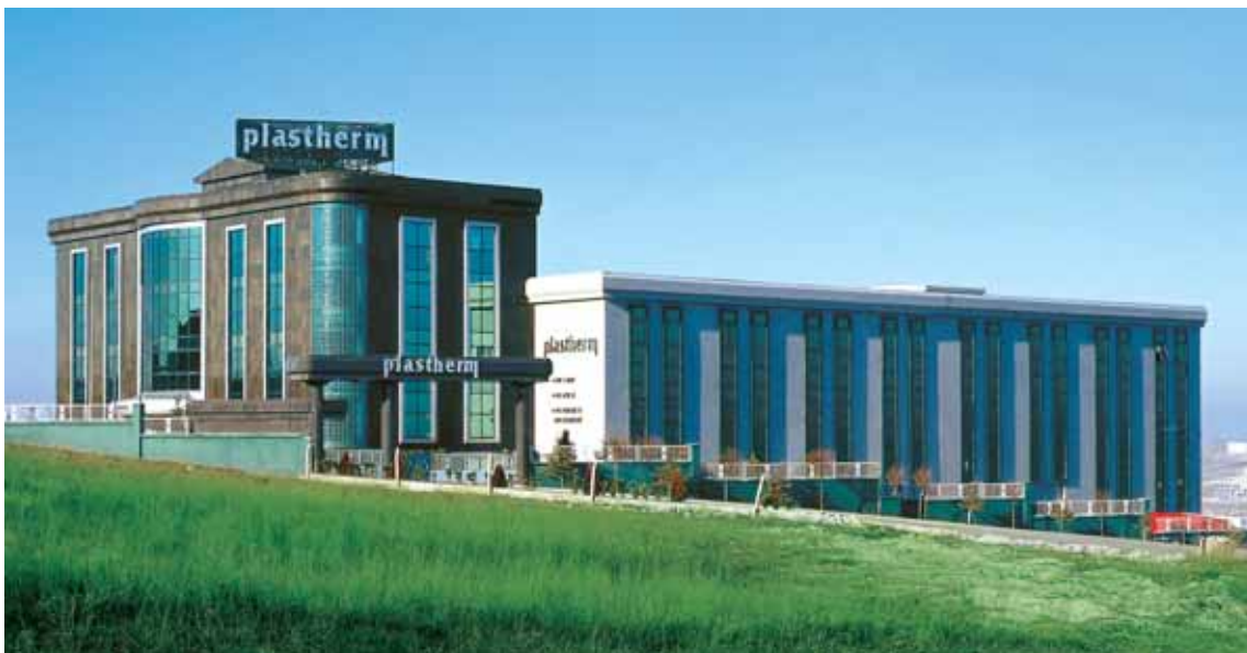
A view of our production plant
