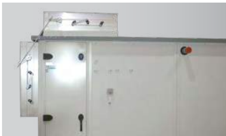
Coupling rod for dampers
