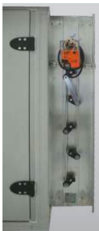
Internal or external damper actuator
