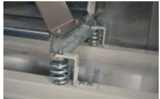
Spring anti vibration mounts
