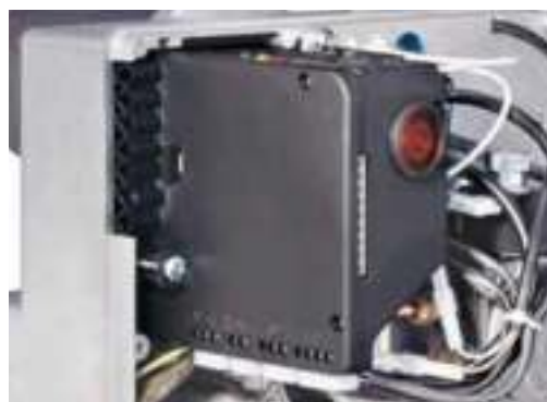
Control box fitted with ignition transformer
