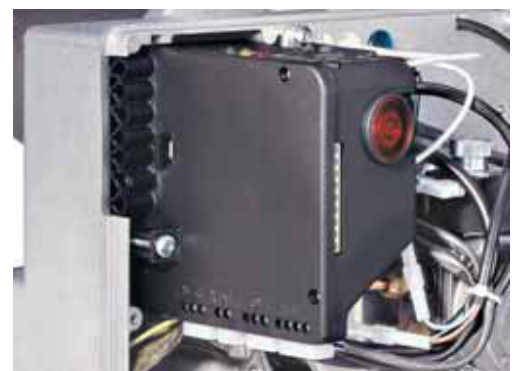
Control box fitted with ignition transformer
